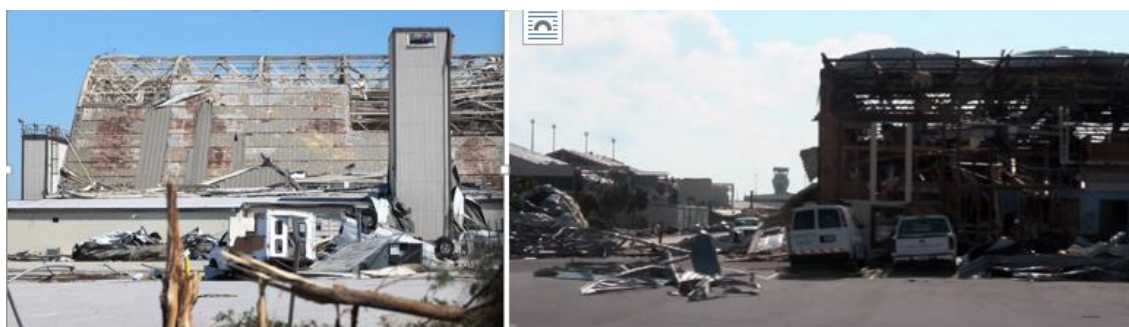
A damaged airplane hangar is seen on the grounds of Tyndall Air Force Base, Fla., after Hurricane Michael passed through the area on 12 OCT
